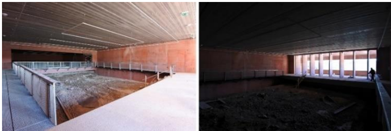
Figure 8-9: The interior of the exhibition space during the construction (courtesy by the Narmer Architecture Studio Budapest)
