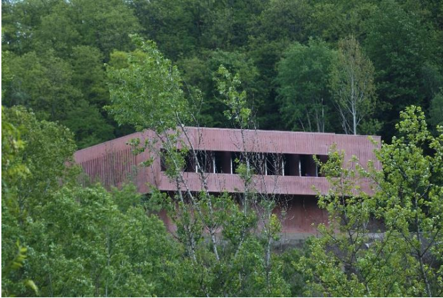
Figure 10: The protective building in the landscape (courtesy by the Narmer Architecture Studio Budapest)
